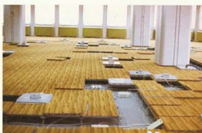
ACULEUM, office building in Frankfurt/Niederrad, Germany where 28.000 sqm of MERO Access Floor type 4 were installed. Design and installation: J. S. K. P&W
