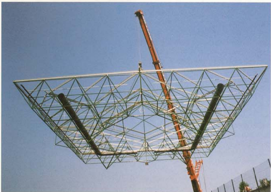
Lifting of space frame structure 24 x 24 m with pre-installed air ducts
