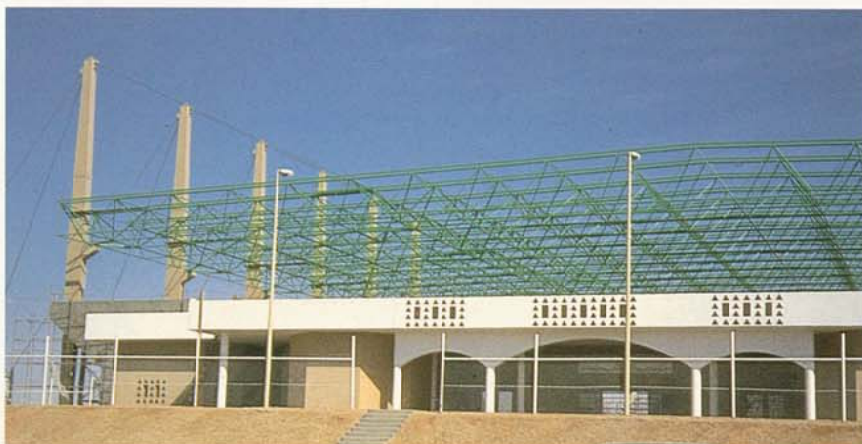
Lifting of space frame structure 24 x 24 m with pre-installed air ducts
