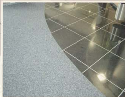
Creative cut at the transition from stone tile to carpet covering.
