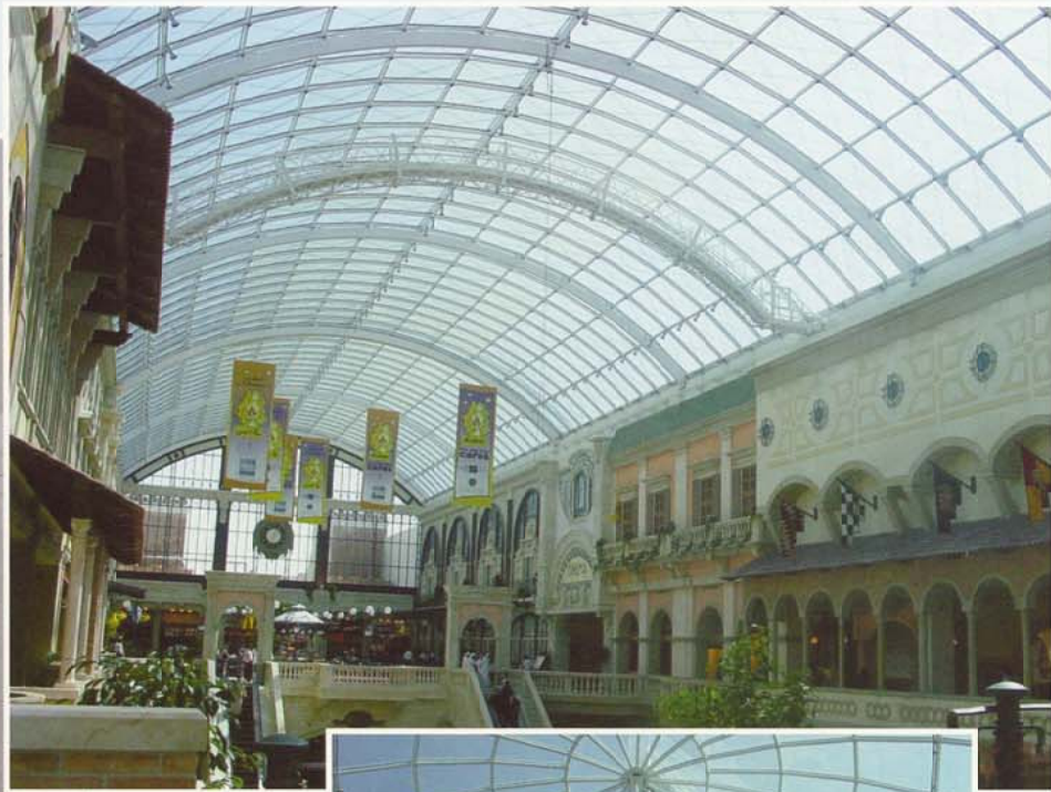
Sahara Center, Sharjah (UAE) Project Management: Al Nibras Engineering, Dubai (UAE)
