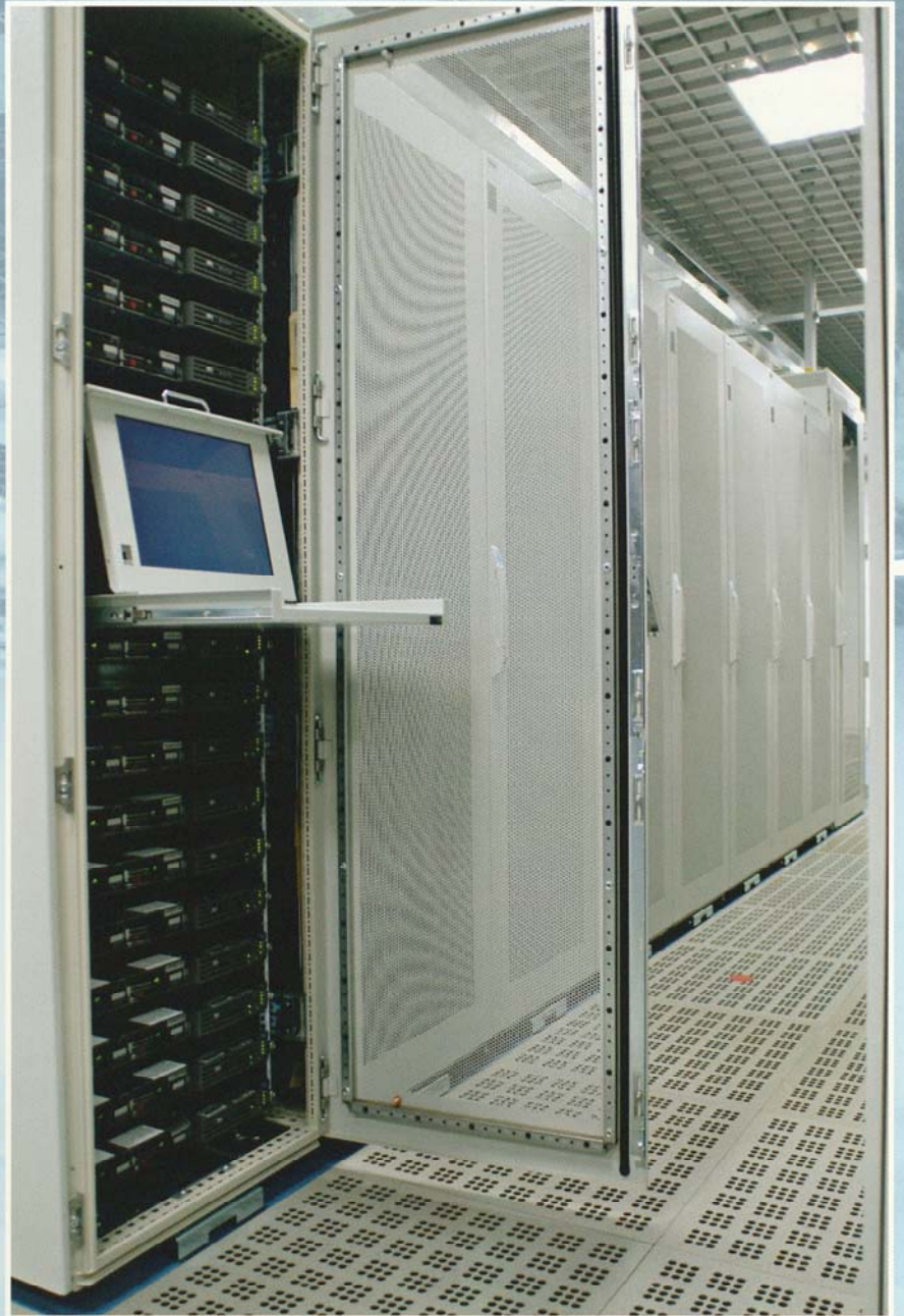
Cool air flows into the rooms through ventilation panels with gradual air flow control
