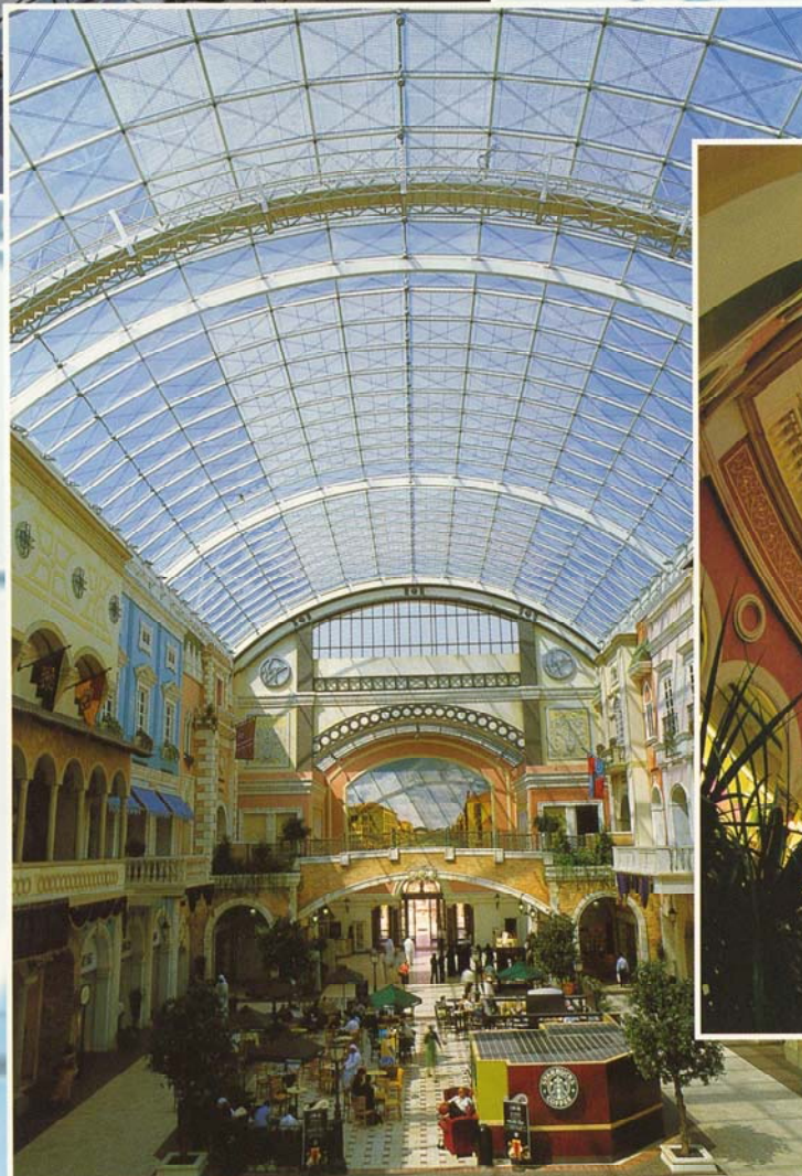
MERCATO, Dubai Transemirates Contracting, Dubai
